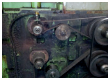
Fig. 3. Belt drive before reconditioning.
